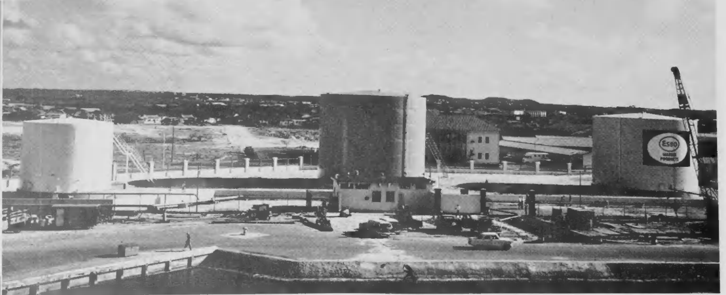
THE TERMINAL building is flanked by three storage tanks which have a total capacity of about 50,000 barrels. Three grades of bunker fuels are available to ships calling at Oranjestad Harbor. NA CADA banda di edificio di terminal ta keda tres tanki di almacenaje cu tin un capacidad total di como 50,000 barril. Tres calidad di combustible ta disponible pa bapornan dren-tando haaf di Oranjestad.
